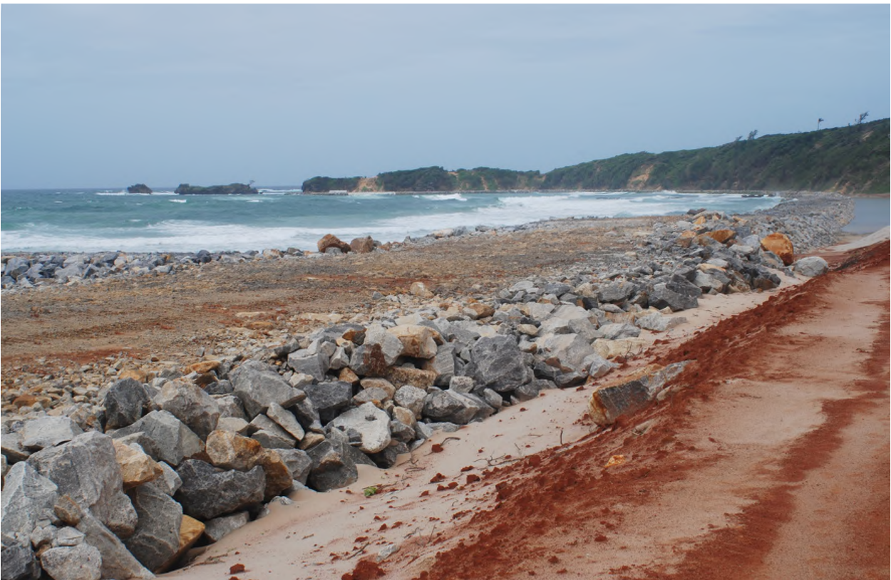
2. Early stages of the port construction.
