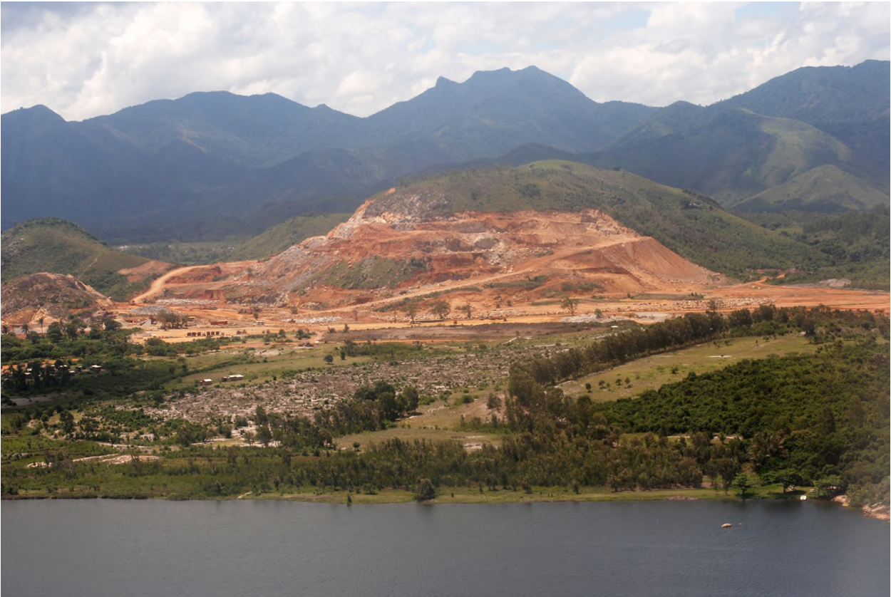
1. View of the quarry site to supply stone for the port, new Mandena road and mine. Reflective roofs of the houses built by QMM for PAPs can be seen bottom right.
