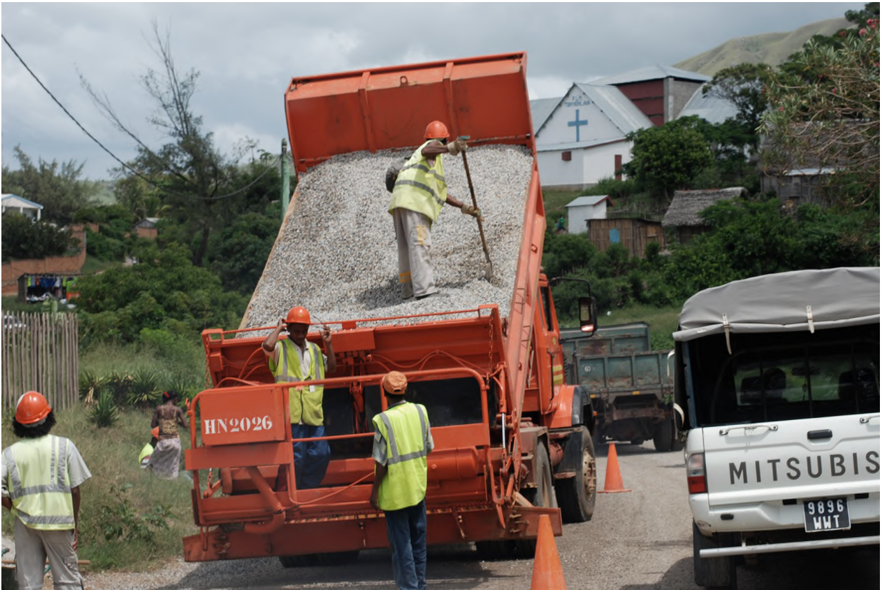
3. Road improvement works in Fort Dauphin by QMM contractor Colas.
